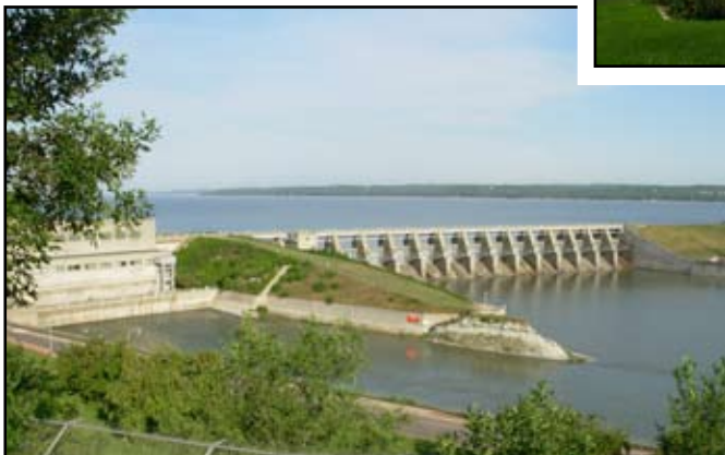
Gavins Point Dam
