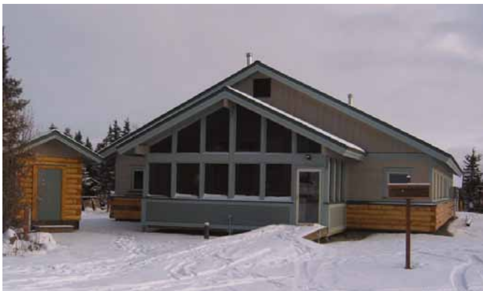
Three 2.5-kilowatt photovoltaic arrays provide enough solar power to run this joint U.S. Fish and Wildlife Service/National Park Service office in Bettles, AK, on most sunny days between March through September. (USFWS)
