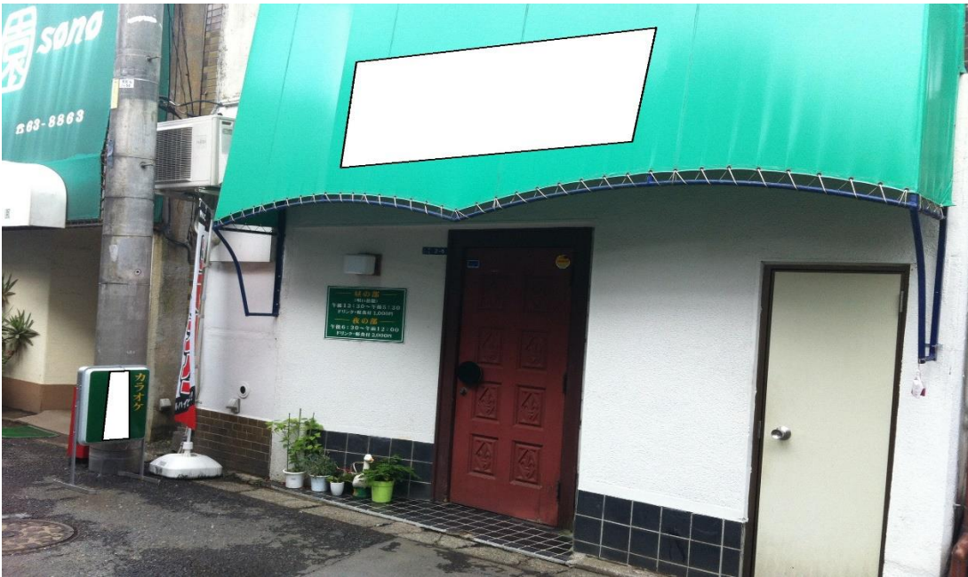
Figure 9: Facade of Sachi. The actual name of the establishment has been blocked out for privacy reasons.
