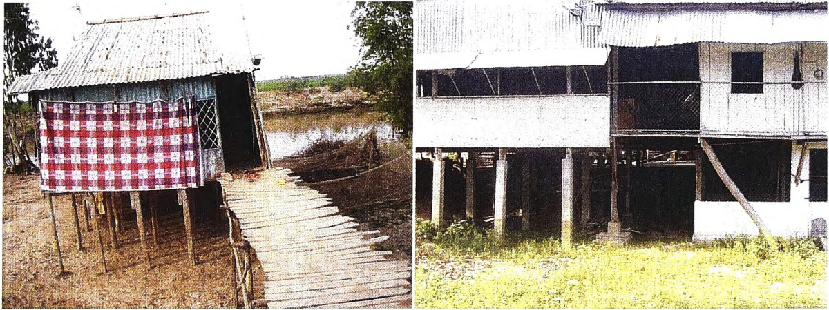
Figure 3. 11: Houses of the poor (left) and of the better-off households (right)
