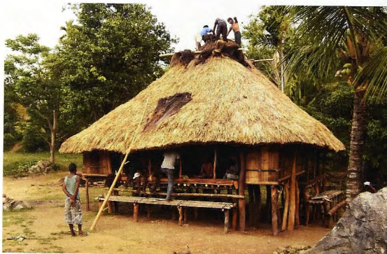
Fig. 7.20 Reconstruction process of a sacred house: final stage.
