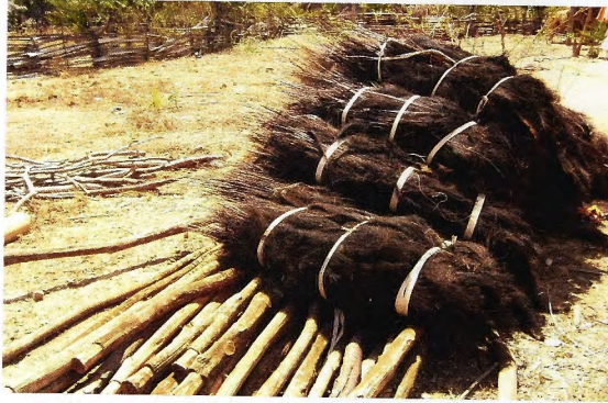
Fig. 7.3 Timber and imperta grass ready to be hand carried to the top of a hill where Larigua house was originally situated.
