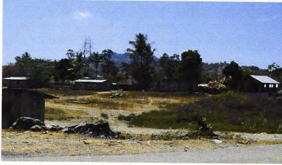
Fig. 5.3 Dilapidated Indonesian-era public housing stands next to thatched housing, Simpang Tiga.
