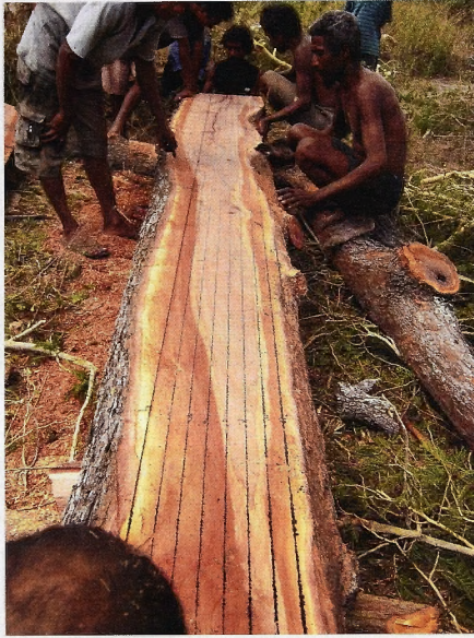
Fig. 7.1 Men and boys preparing to cut wooden planks for Lari'gua house construction.
