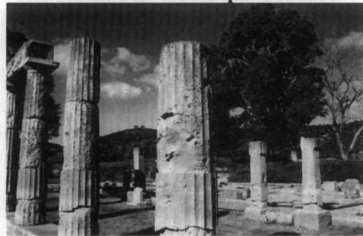
Figure 15 - Different degree of decay on column pieces
