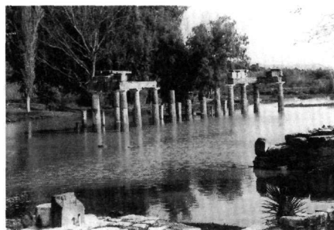
Figure 27 - Brauron monument (26/11/2005) Erasinos flooded after strong rainfalls
