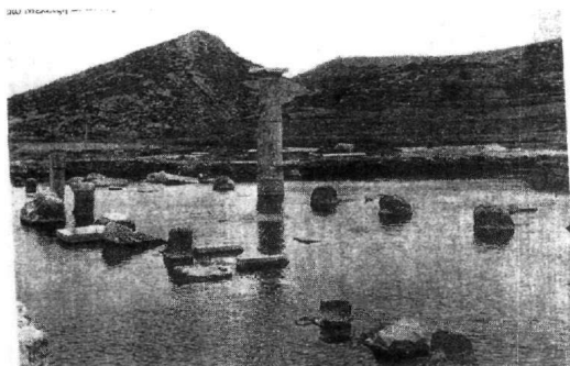
Figure 26 - Brauron monument before the restoration works (photo by Bouras 1967)
