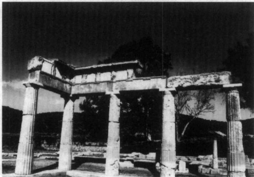
Figure 14 - Different degree of decay on capitals and Calcareous crust development
