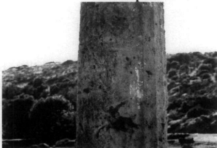
Figure 18 - Intense decay form on sandstone type III
