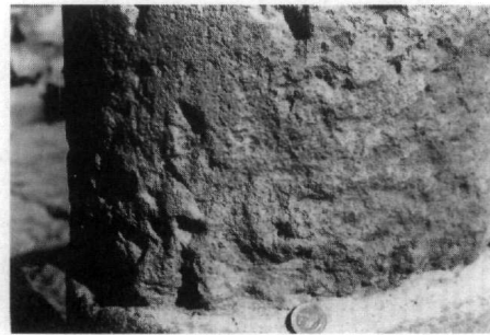
Figure 19 - decay form on sandstone type I
