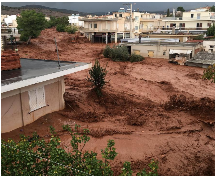
Fig. 7: The flood flow in the residential fabric of Mandra.
