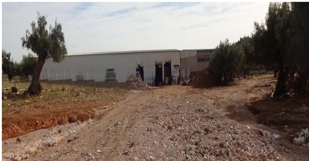
Fig. 5: Photograph of the Soures streambed which shows the existence of a massive building across the flow of the stream.
