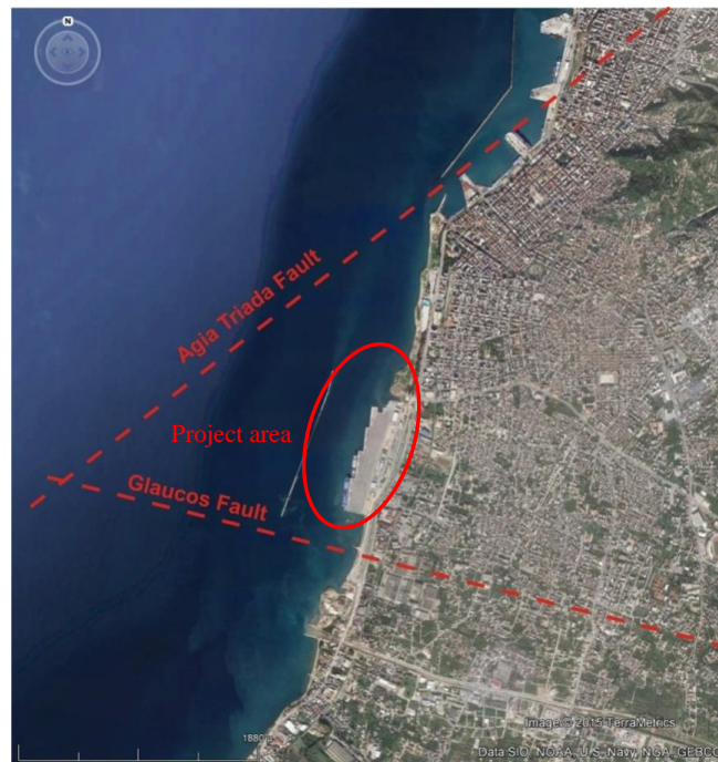
Figure 2 - The location of the "Agias Triada" and "Glaucos" faults in relation to the New Port of Patras.
