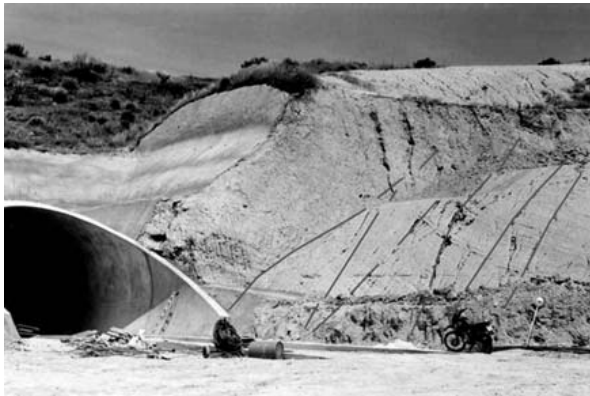
Photo 1: Southern portal of tunnel SB (left branch). The two units (Upper and Lower ones) are distinguished, due to color and structure. Their continuity is interrupted by faults that considerably change dipping.
