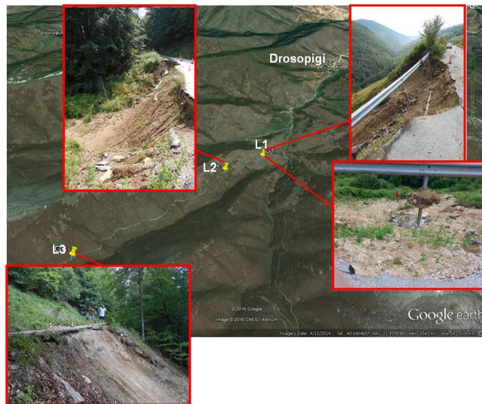
Figure 5 - A general view of Vitsi landslides (L1, L2, L3).
