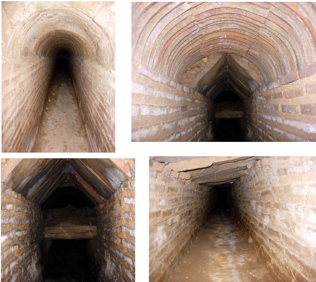
Fig. 3. The inclined gallery of the Hadrianic aqueduct at the Olympic Village; various types of support with standardized bricks are shown (Horne, 2009).
