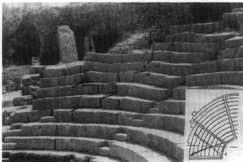
Fig. 6. Photograph of the 3 rd century BC terraced seating (auditorium) of Butrinti Theatre. Deformed construction and especially open fissures are shown by arrows at the western side of the auditorium. Right down corner: the sketch of the diagonal shear cracks.
