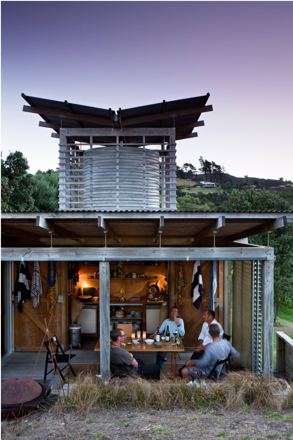
Figura 28 Herbst Bach – Hersbt Architects. Jackie Meiring
