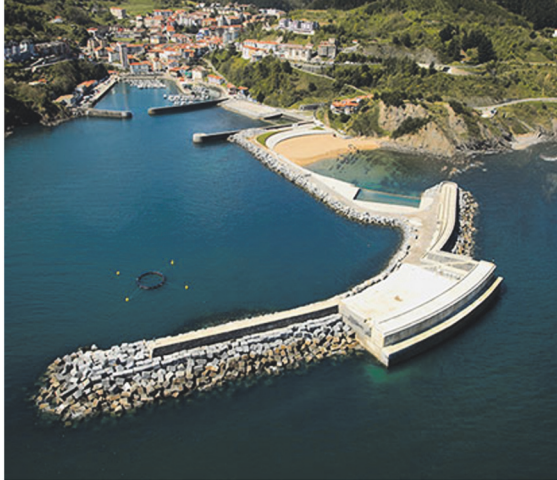
FIGURE 1: The OWC power plant of Mutriku.
