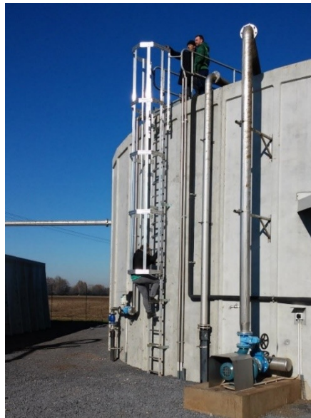
Figure 16 SBR tank. In the Figure a) it is possible to see the pipe that connect the SBR's outlet with a storage tank, where the effluent is collected and stored for further utilization. In Figure b) a particular of inlet and aeration system.
