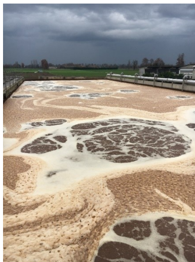
Figure 14 a) the recirculation apparatus, b) mixing tanks where denitrification occurs and b) aeration phase for nitrification process.
