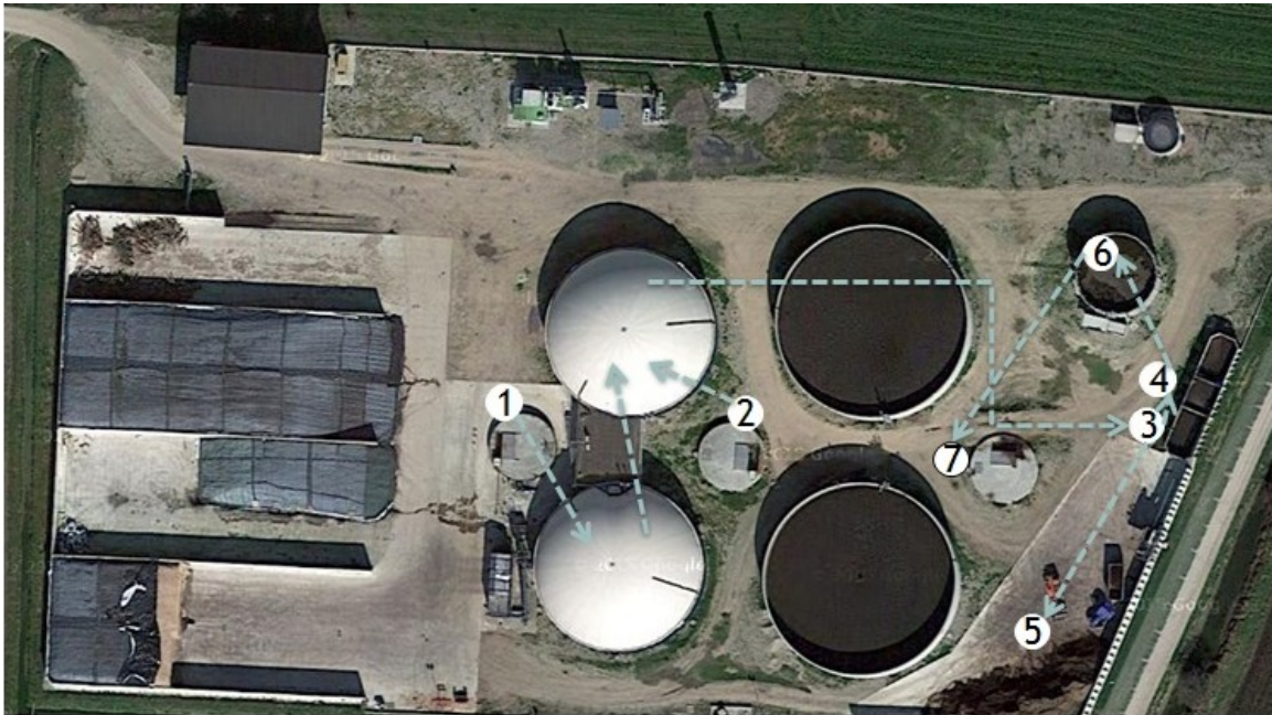
Figure 18 Overview of Plant NA: 1 and 2 are two inlet points, where the slurry is charge and enters in the plant; 1,2: are two inlets points; 3: storage of digestate after AD process; 4: liquid fraction of digestate; 5:solid fraction of digestate; 6 SBR; 7 final storage tank.
