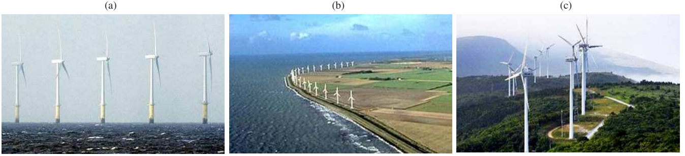
Fig. 1. Different wind farm environmental conditions profoundly influence the production and the complexity of the power prediction for (a) offshore wind farms, (b) nearshore wind farms affected by periodic breezes, and (c) wind farms with complex orography and nearby hills.
