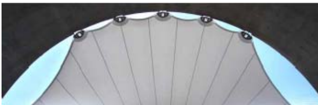
Fig. 5: Point-type supports [1]
