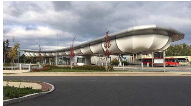
Fig. 3: Bus station in Bruntal, 2018
