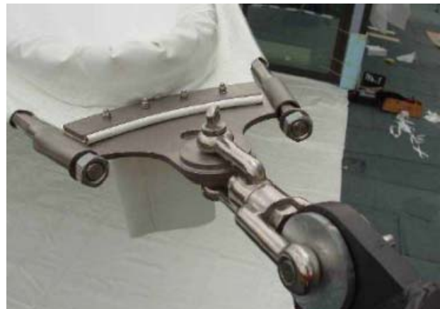
Fig. 8: Connection between the corner plate of a membrane and the joint plate [1]
