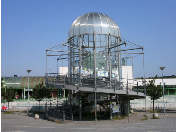
Fig. 3: An example of an inadequately designed ramp that does not allow separate barrier-free use (slope and shape) - Prague - Cerny Most (author: Alzbeta Bilkova, 2013).
