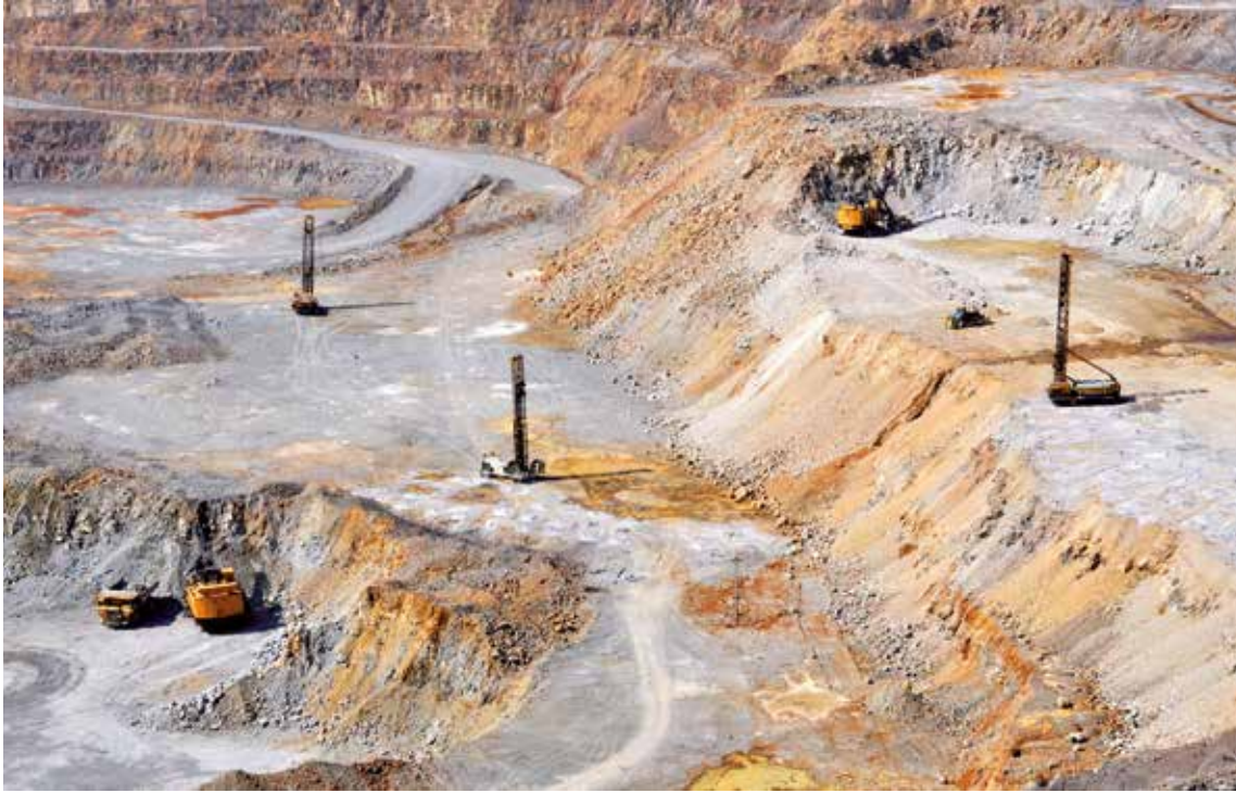
2.1 > Mineral ores for metal production are extracted from huge open-cast mines such as the Dexing copper mine near the eastern Chinese city of Shangrao. The excavators are working their way deep into the earth.
