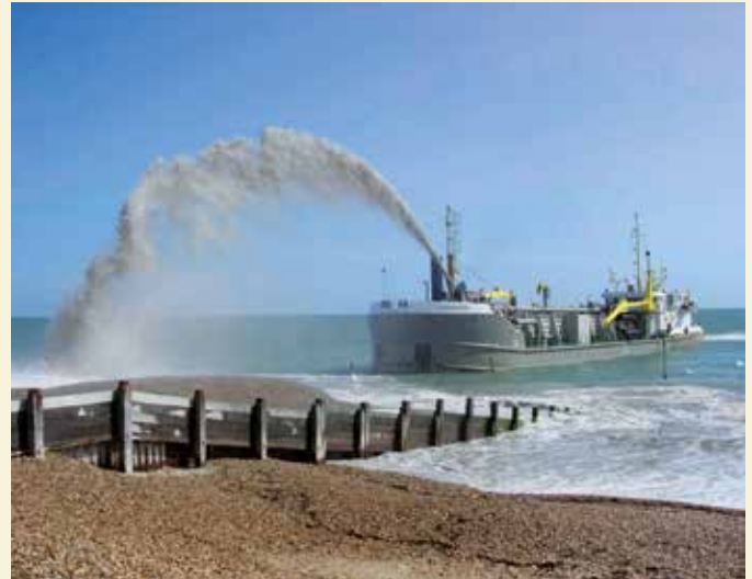
2.9 > The sand-water combination is pumped from the ship onto the beach using the "rainbow method".
