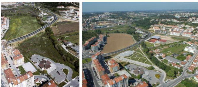
Figure 7. Aerial view over the DPI sportive area before (left) and after the intervention (right). Photographic credits: Polis Leiria.
