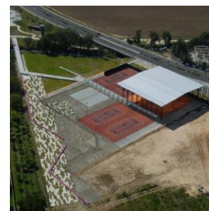
Figure 16. Aerial view over their construction park area. Photographic credits: Leiria Polis
