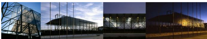
Figure 13. Acoustic barrier and wind guard panel for the game fields protection. Photographic credits: Catarina Costa Cabral
