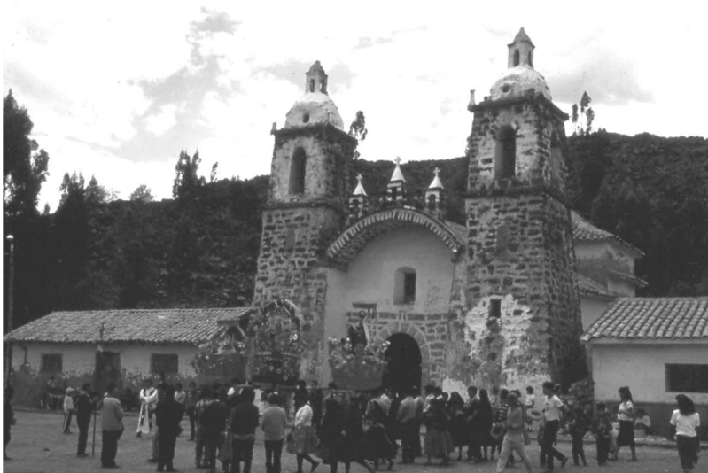
Figure 6. The church at Raqchi during the celebrations for San Miguel (1991) (note the repair to a crack in the right-hand tower). © Photograph: Bill Sillar.
