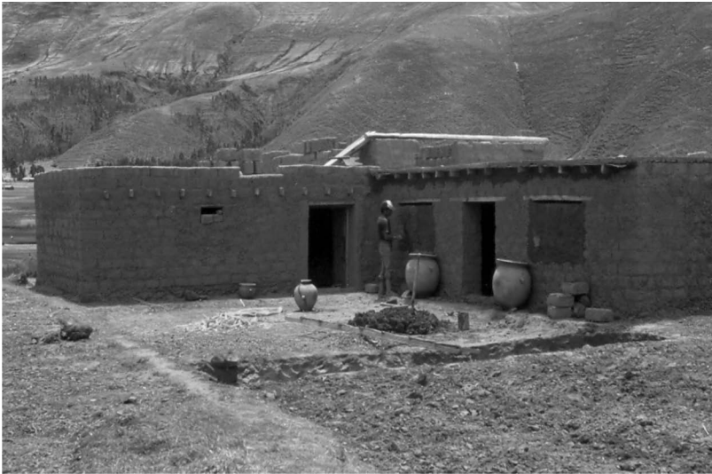
Figure 3. Maximo Amaru during construction work on his house in 1985 (in the process of blocking the window openings with adobe bricks). © Photograph: Bill Sillar.
