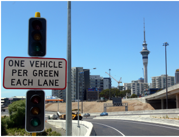
(a) Ramp-metering. Photo by Benpaul12 at English Wikipedia (Public domain), via Wikimedia Commons.
