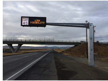
(b) Variable Speed Limit. Photo by Oregon Department of Transportation (CC BY 2.0).
