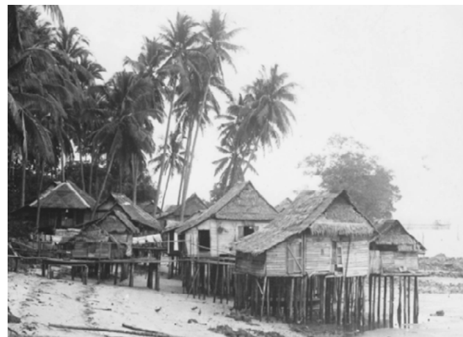
Figure 6: Attap dwelling with attap roof and walls in Malay village
