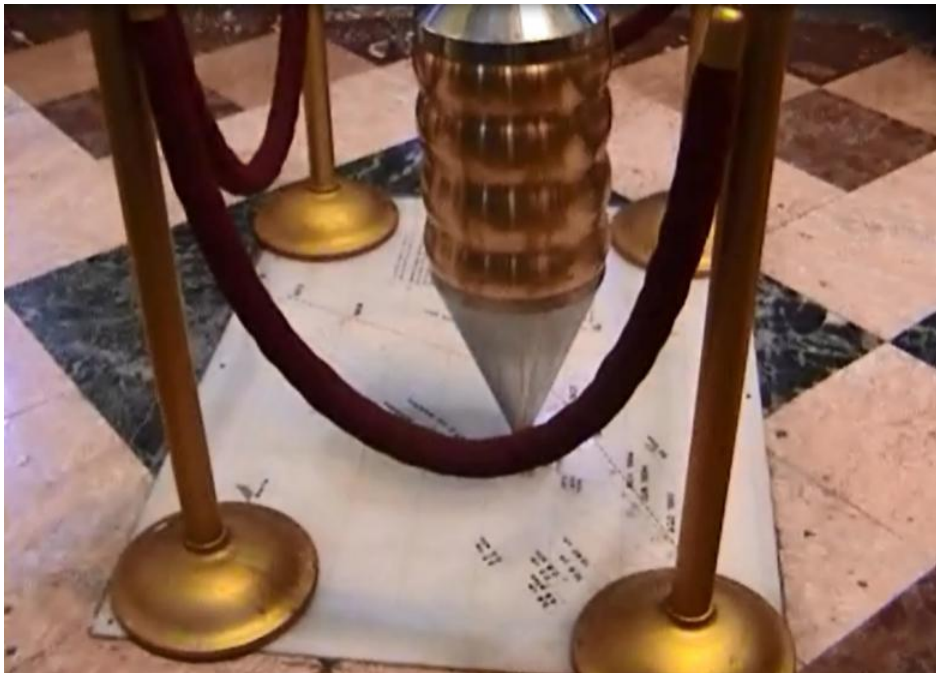
Fig. 6. 6. Uneven sinking of a building structure due to groundwater extraction, as illustrated by the displacement of a plumb-bob in the central basilica in Mexico City (author's photo from 2001).
