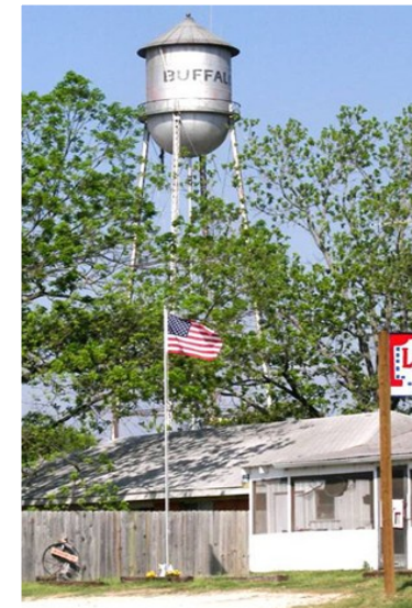
Figure 1.2. Buffalo water tower (Photo credit: Barclay Gibson)
