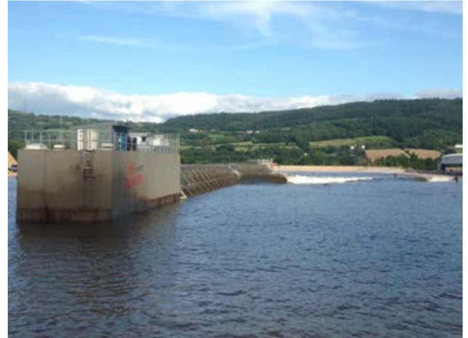
Fig.02 The wave-generating mechanism at Surf Snowdonia, Wales, viewed from its western end. The wave is situated in a re-purposed reservoir and is created by a submerged engine which runs across a track in the centre, pushing a wave outwards on either side. David Whyte.
