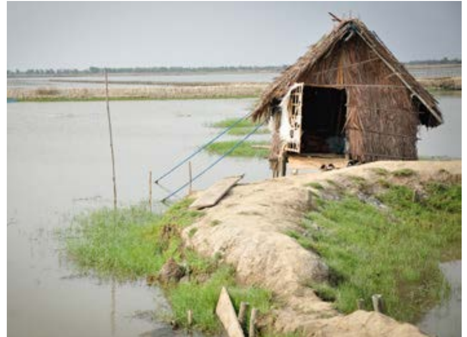
Dwellings commonly found in rural areas are called kutcha and pucca. Kutcha homes are typically made of earthen materials like mud brick, bamboo, timber and plant material. The roofs are often hatched with grasses fastened to a bamboo structure. These earthen materials are relatively economical and readily available to local farmers. These simple, natural materials create climate controlled spaces that are cool in the heat and warm in the winter without the use of expensive materials and unavailable technology.
