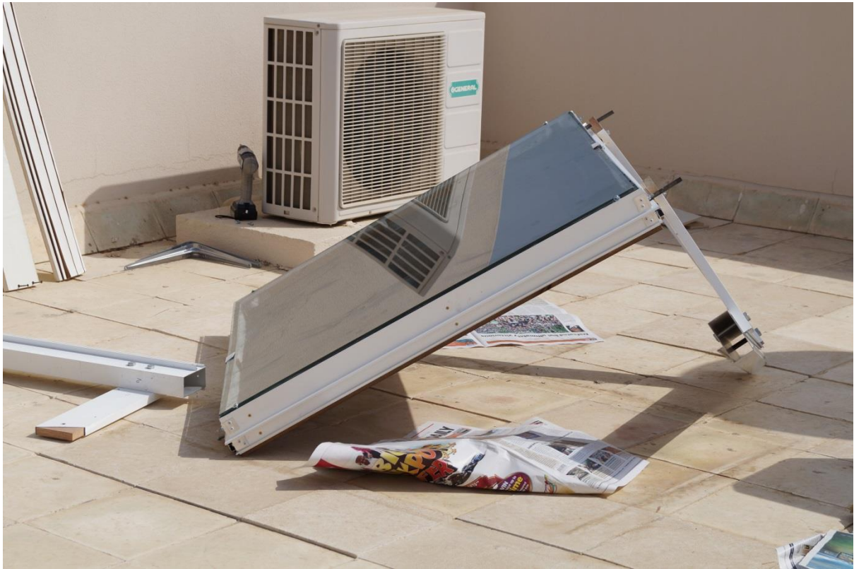
Photo 4.7 Rooftop Assembly in Progress
