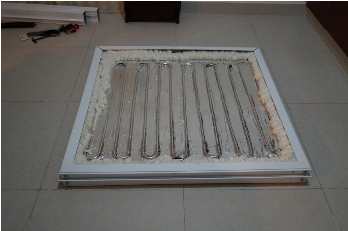
Photo 4.4 Edge Insulation Completed
