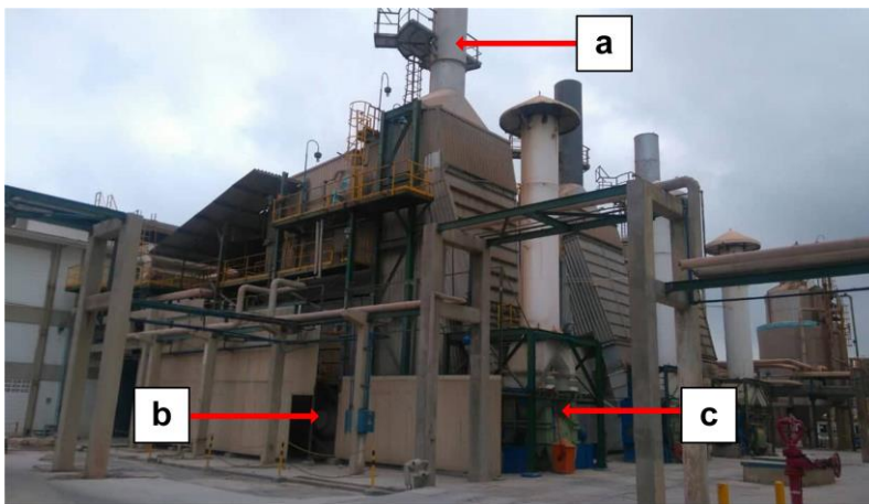
Figure 2. Steam generator main components (a) smokestack, (b) gas burner, and the (c) water supply.
