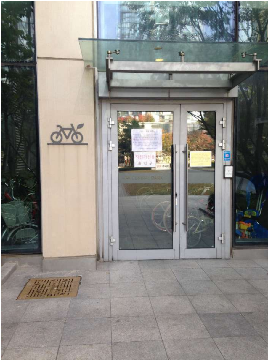
Figure 101 - Sharp II images, Songdo 1st phase construction (source: by the author 2015)
