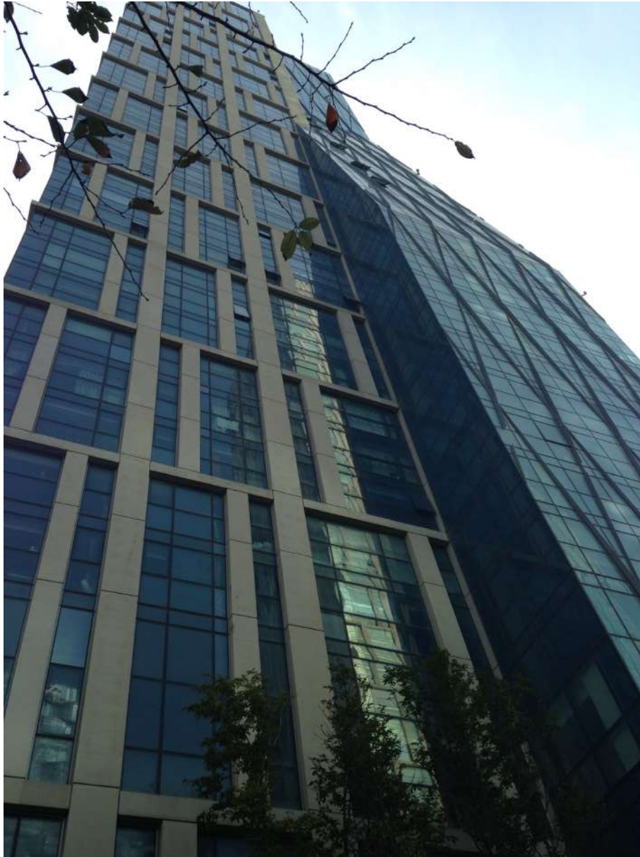
Figure 102 - Sharp II images, Songdo 1st phase construction (source: by the author 2015)
