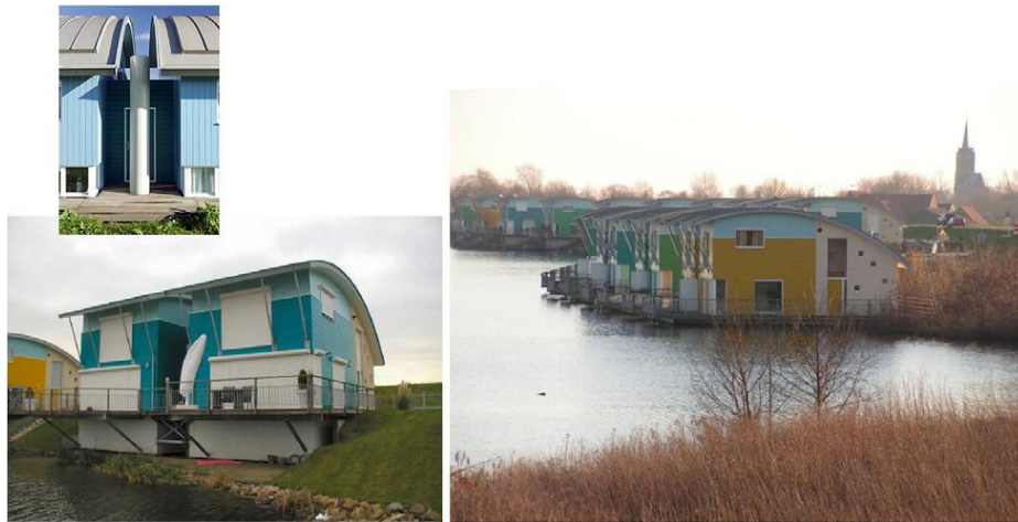
Figure 4 – Amphibious housing built upon resilient dikes in Holland. Source: (Dura Vermeer case study in , Robinson and Hamer, 2009)
