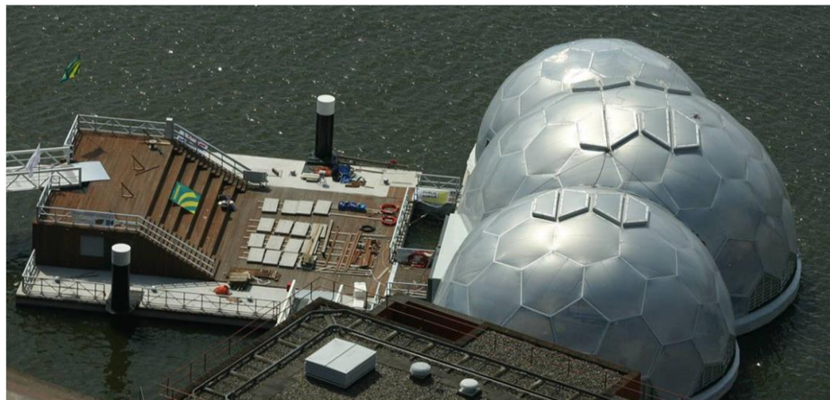
Figure 5 – Floating Pavilion of the Delta Sync and Dura Vermeer, one of the seven projects of the Rotterdam’s climate change adaptation strategy. Source: Author’s photograph
