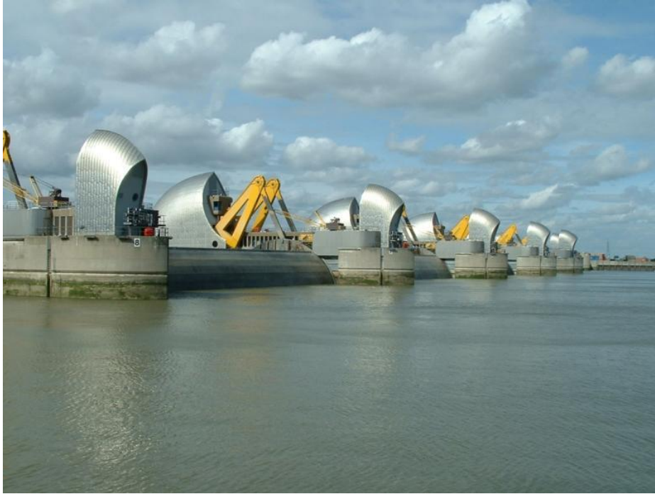
Figure 7 – Water level control in London by the Thames Barrier. Source: Andy Roberts 2004
