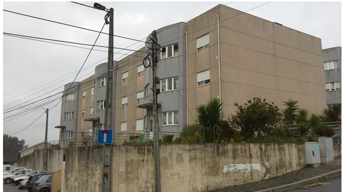
Fig. 1. Photograph of the studied building.
