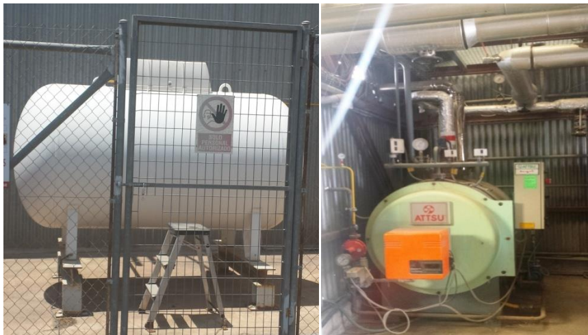
250 Figure 4. The propane gas-fired tank (on the left) and the gas boiler (on the right)
