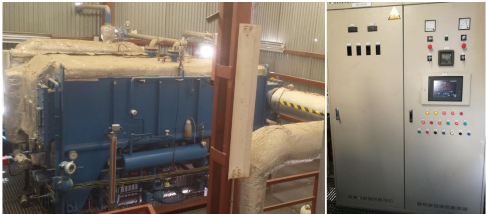
188 Figure 2. DEAHF LiBr-H 2 O facility at the PSA on the left and the programmable logic 189 controller on the right 190
