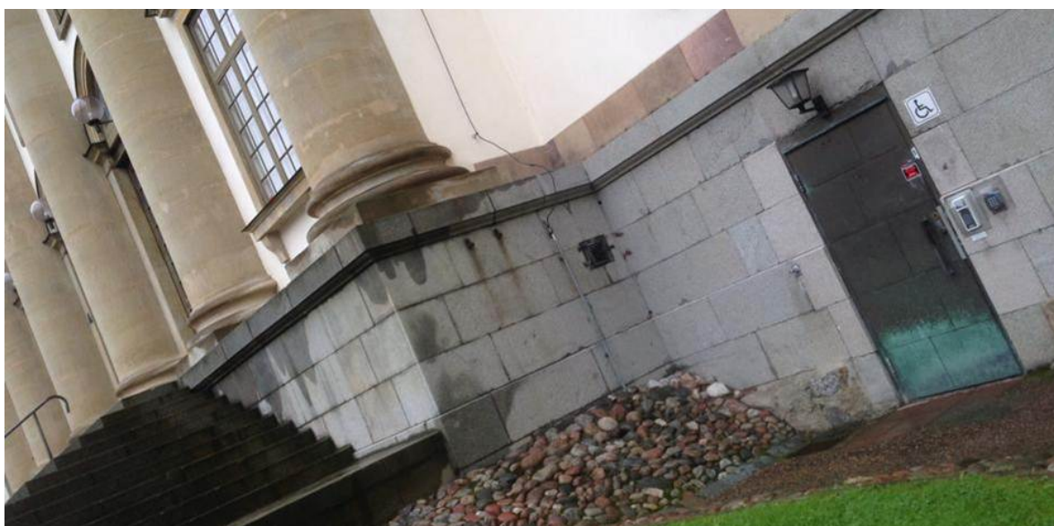
Figure VII Wheelchair entrance in comparison to a lavish main entrance
