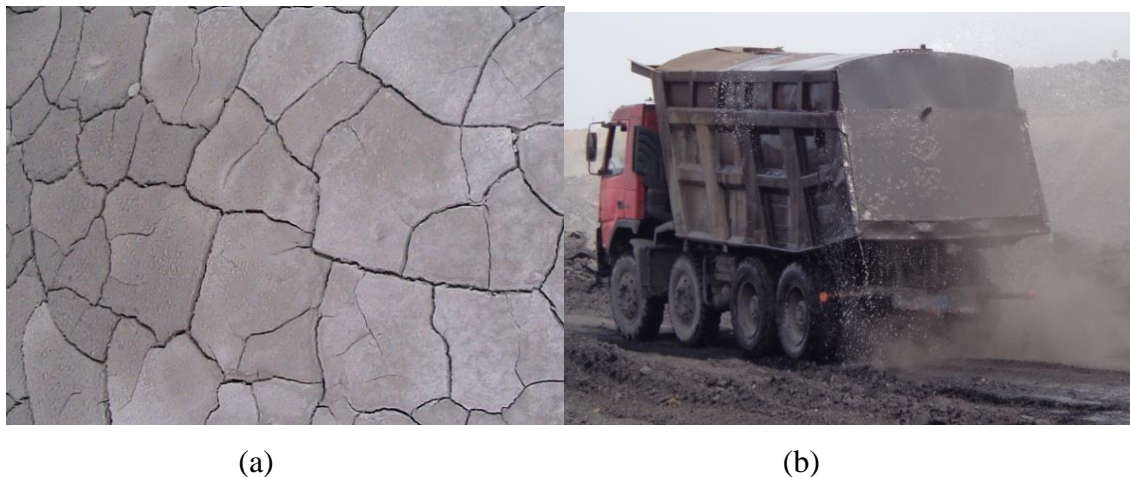
Figure 6.1: (a) Surface crack of a typical mine overburden, (b) Temporary stabilization of dispersive soil by a sprinkling of water.
