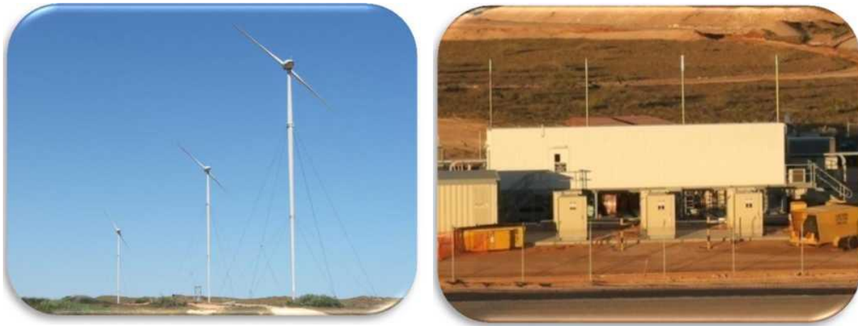
Fig. 4: Coral Bay, Wind/Diesel System Australia
