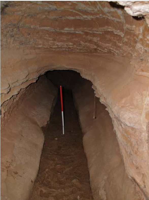
Fig. 13 The unlined tunnel in the qanat at Bureta, Zaragoza.
