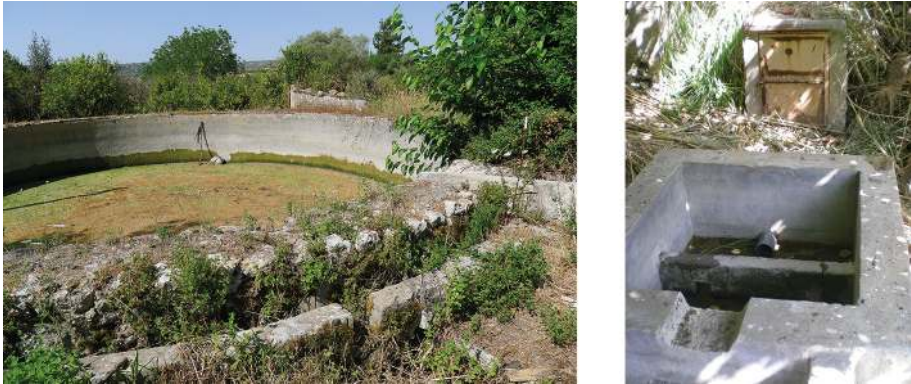
Fig. 2 The irrigation system: Fig. 2a: on the left, private reservoir for storing irrigation water. Fig. 2b on the right, Regulatory tank of irrigation, under the supervision of Genio Civile.
