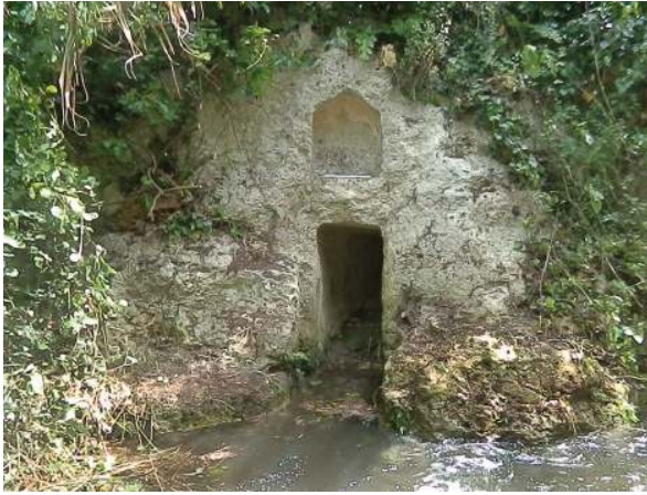
Fig. 3 The Ciccio niche and water intake.
