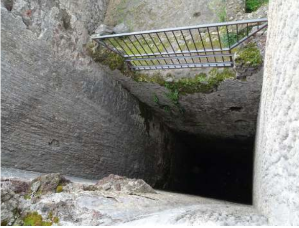
Fig. 7 An ideal deep rectangular shaft for a sizeable bucket-chain in Pompeii, the main installation for the Stabian Baths. The carbonate incrustations can be clearly seen along the left side wall. The original wheel driving the installation was positioned in the room behind the modern fence. The onset of the arc, visible in the back wall of the shaft, held the bucket chain installation.
