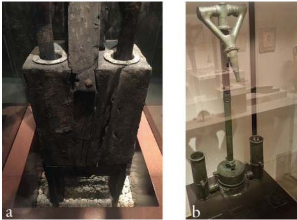
Fig. 3 a) Wooden force-pump found in Bertrange, Luxembourg. The pump dates back to AD 270 and was found in the Roman fort. The original remains are in the National Museum of History and Art in Luxembourg. b) This example of a force-pump is made of bronze and was used in the Sotiel Coronada copper mine in southwest Spain, either as a fire-extinguisher or to spray cold water on rocks to fragment them. This force-pump dates back to the Imperial Roman period and is housed at the National Archaeological Museum in Madrid.
