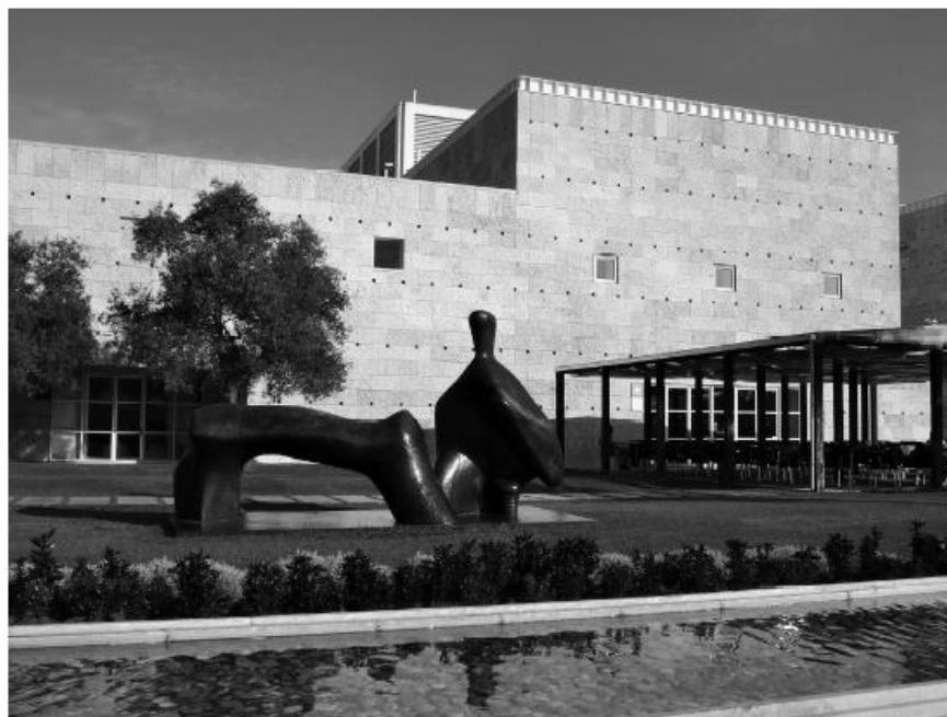
Figure 16.4 Centro Cultural de Belém/Belém Cultural Center (Lisbon)
