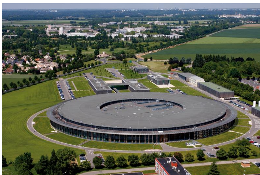
Figure 1.6 - SOLEIL synchrotron. Saint-Aubin, France. (adapted from - http://enygf2015.org/program/technical-visits/saclay/ )
