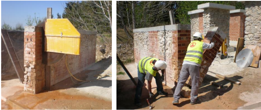
Figure 3. Sectioning the wall specimen M1 [3].
