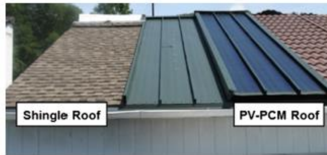
Fig. 4.42. PV-PCM roof [193]
