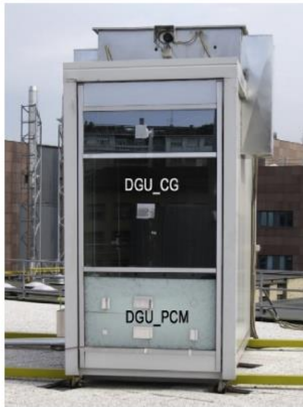
Fig. 4.26. Experimental test cell with the two glazing systems (DGU_PCM and DGU_CG) [144]
