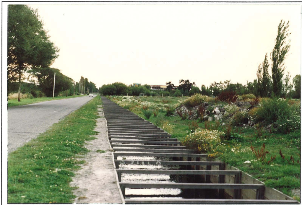
Figure 4.1. Drain leading from Travis swamp.
