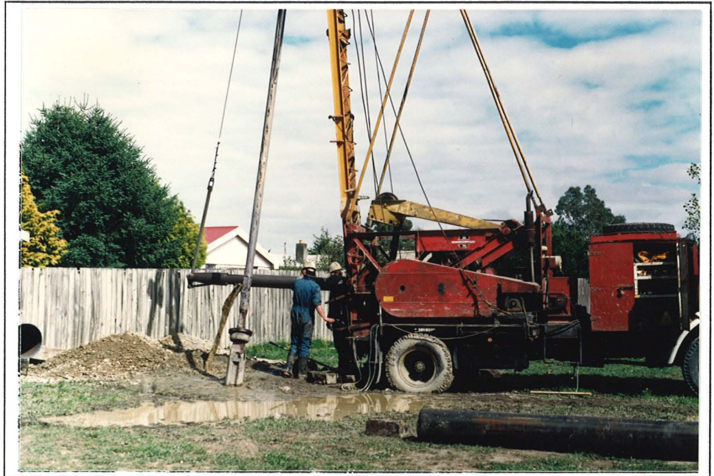
Figure 4.33. Well being sunk in Woodbury Street, Avonhead 1989.
