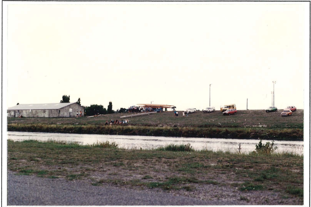
Figure 4.28. Kerr's Reach. The cut from the diversion became fill for a grandstand.
