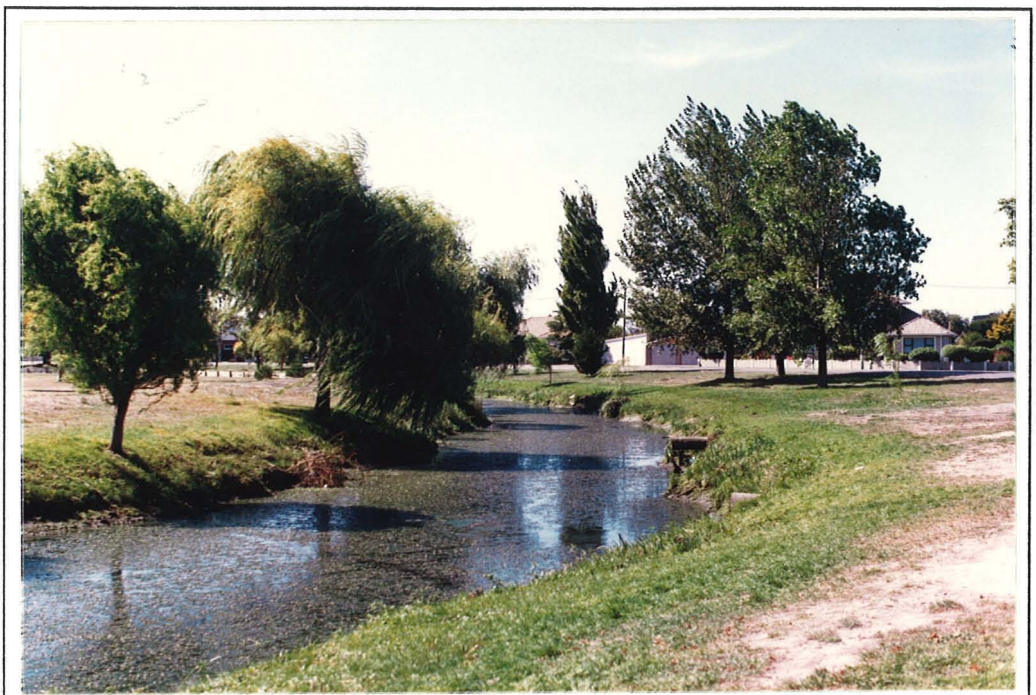
Figure 4.29. The sluggish portion left after Kerr's Reach diversion.
