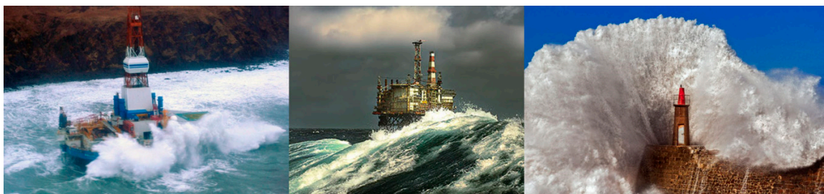
Figure 2. Some examples of wave run-up in different gravity structures occurring after violent wave impact. As can be observed, the crown elevation of the structures is not always designed at a level protected enough from wave impact actions. Source: The New York Times and own collection.
