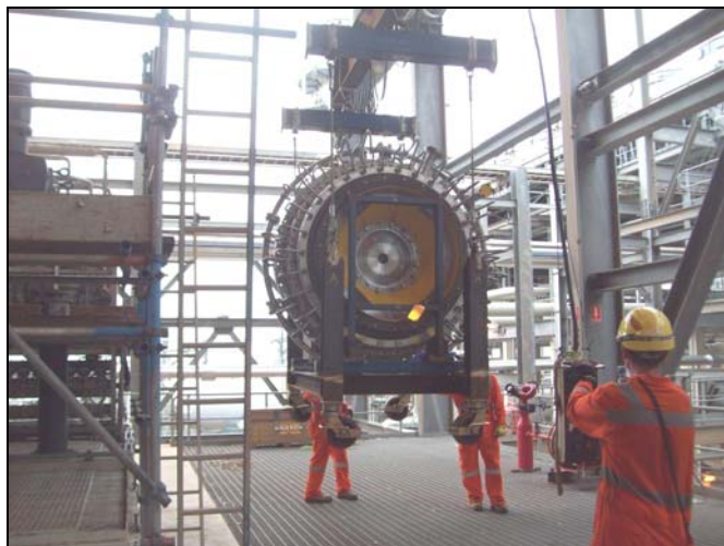
Figure 42. High Speed Power Turbine Being Moved into place for Installation.
