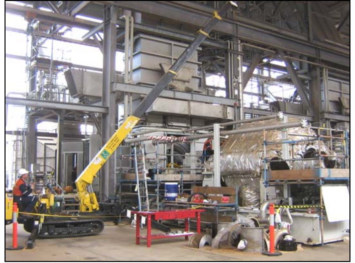
Figure 36. Propane Compressor Tertiary Seal Change out Activities.
