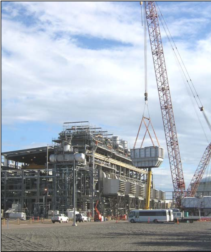
Figure 35. Change Out of OTSGs.
