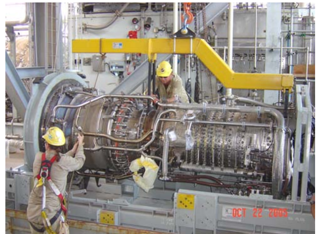
Figure 7. LM2500+ Gas Generator Being Installed.
