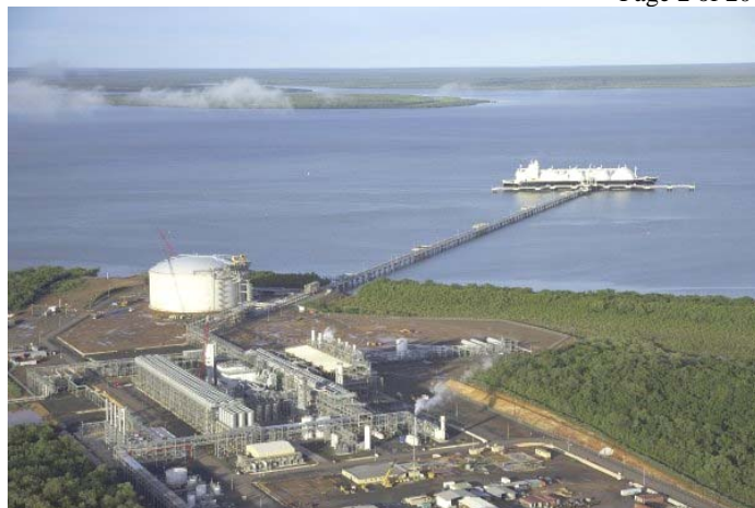
Figure 2. Aerial View of the 3.7 MTPA LNG Plant.
