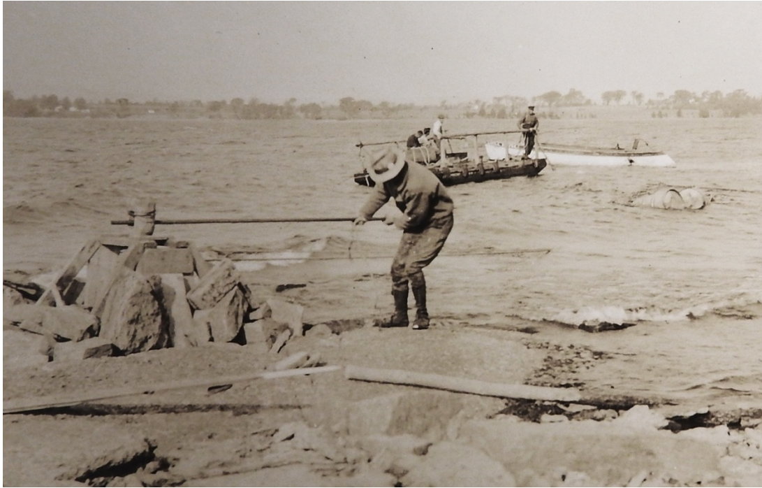
Fig. 4-4. The homemade winch and raft used for raising the Royal Savage remains. Reprinted from Hagglund Collection [NHHC, Folder RS-056] with permission from from NHHC, 2017.
