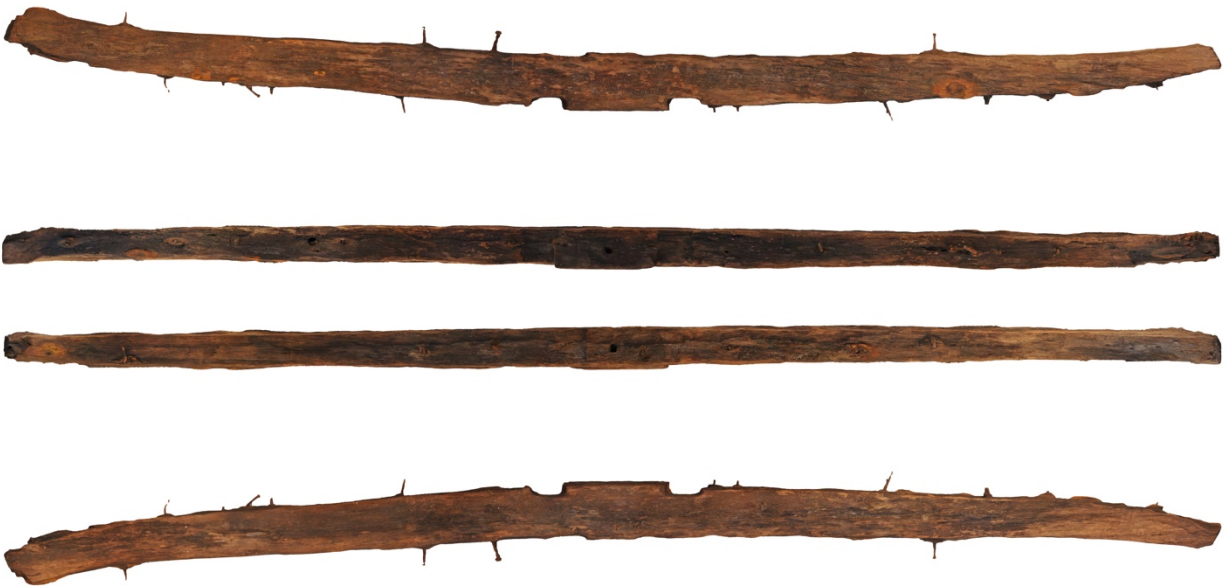
Fig. 7-4. Orthophotos of each face of timber RS-26 extracted from the photogrammetric model.
