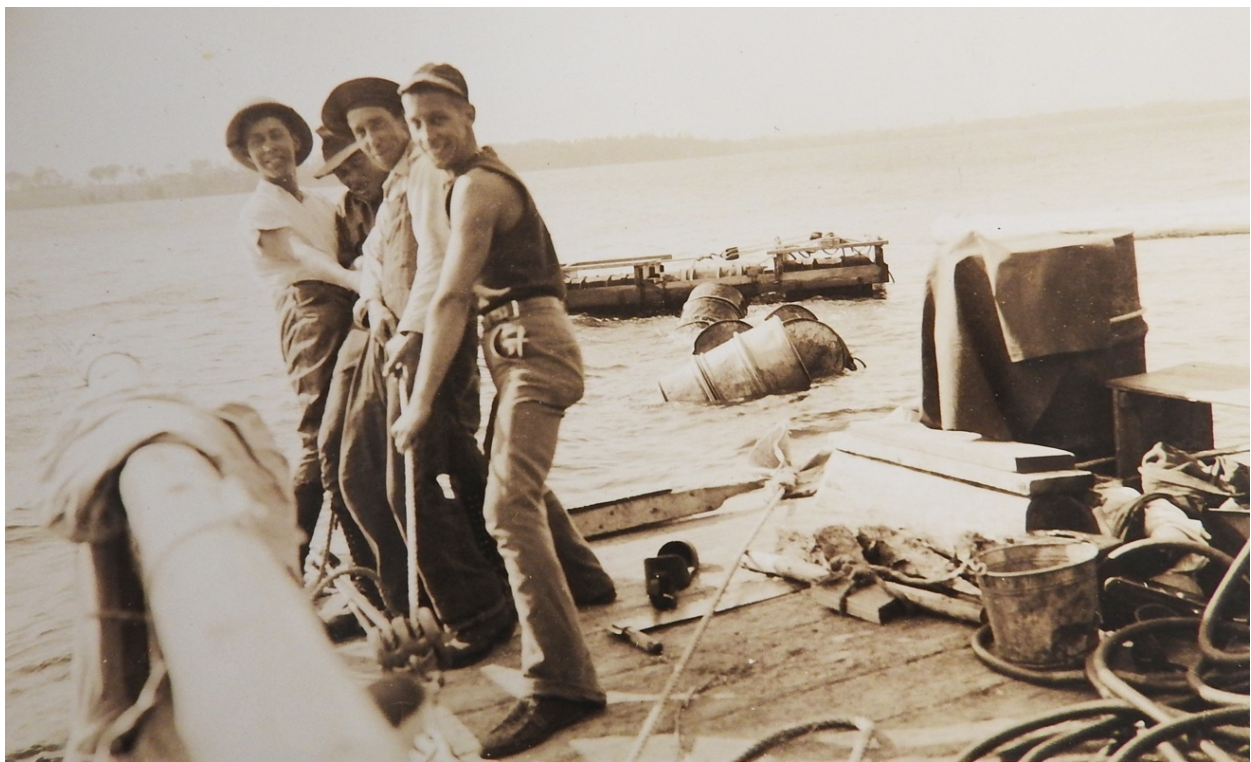
Fig. 4-3. The tar drums that were used to lift Royal Savage . Reprinted from Hagglund Collection [NHHC, Folder RS-056] with permission from NHHC, 2017.
