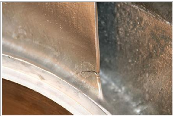
Figure 3: G-2001 old rotor 3 rd stage vane inlet
