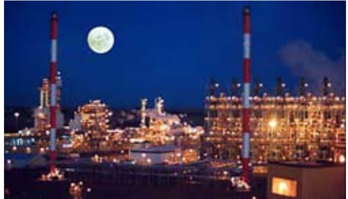
Figure 4. NOVA Chemicals' Joffre manufacturing facility.
