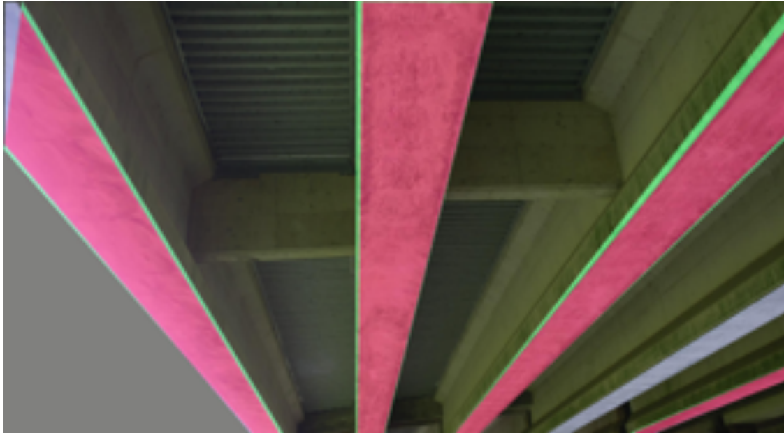
Figure 7.16. Full beam detection of beam flange.
