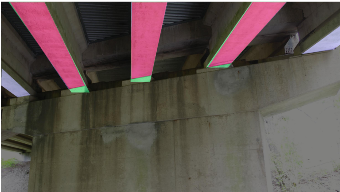
Figure 7.12. Full beam detection of beam flange: Example 1.
