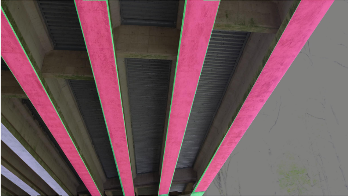
Figure 7.13. Full beam detection of beam flange: Example 2.
