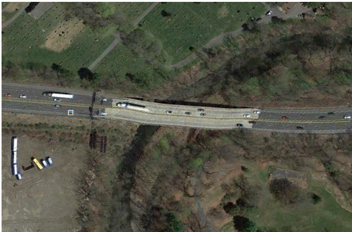
Figure 4.3. Bridge detail: SR 80 (LR 794).
