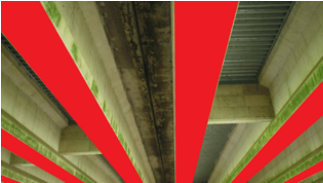
Figure 7.3. Example of manually masked beam flanges.
