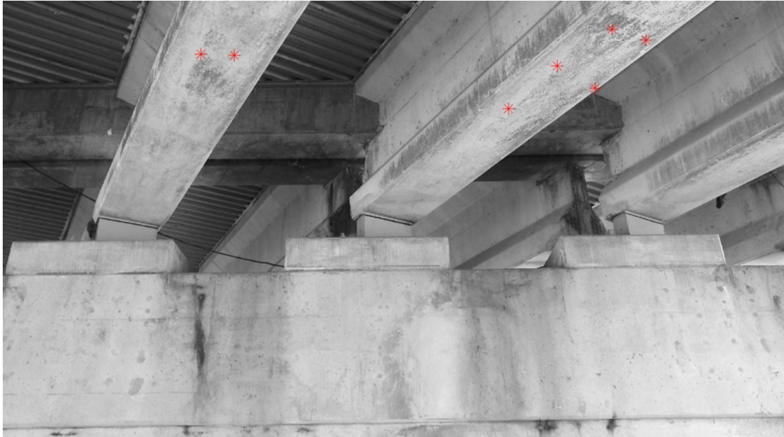
Figure 7.11. R CNN detection of beam flange: Example 4.
