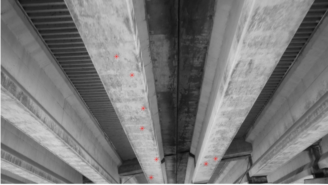
Figure 7.10. R CNN detection of beam flange: Example 3.
