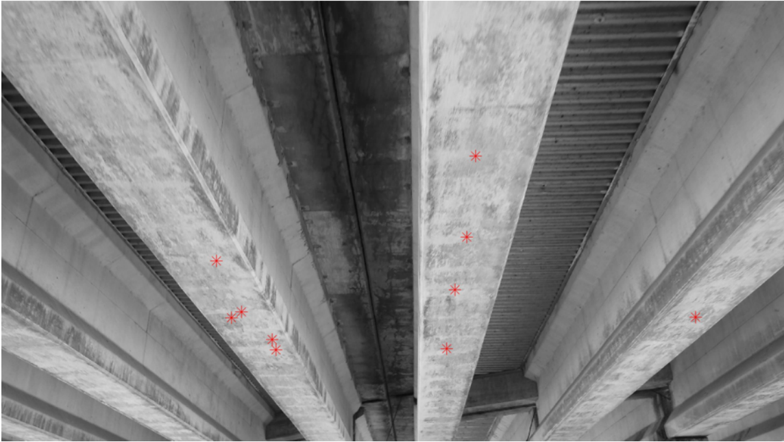
Figure 7.9. R CNN detection of beam flange: Example 2.
