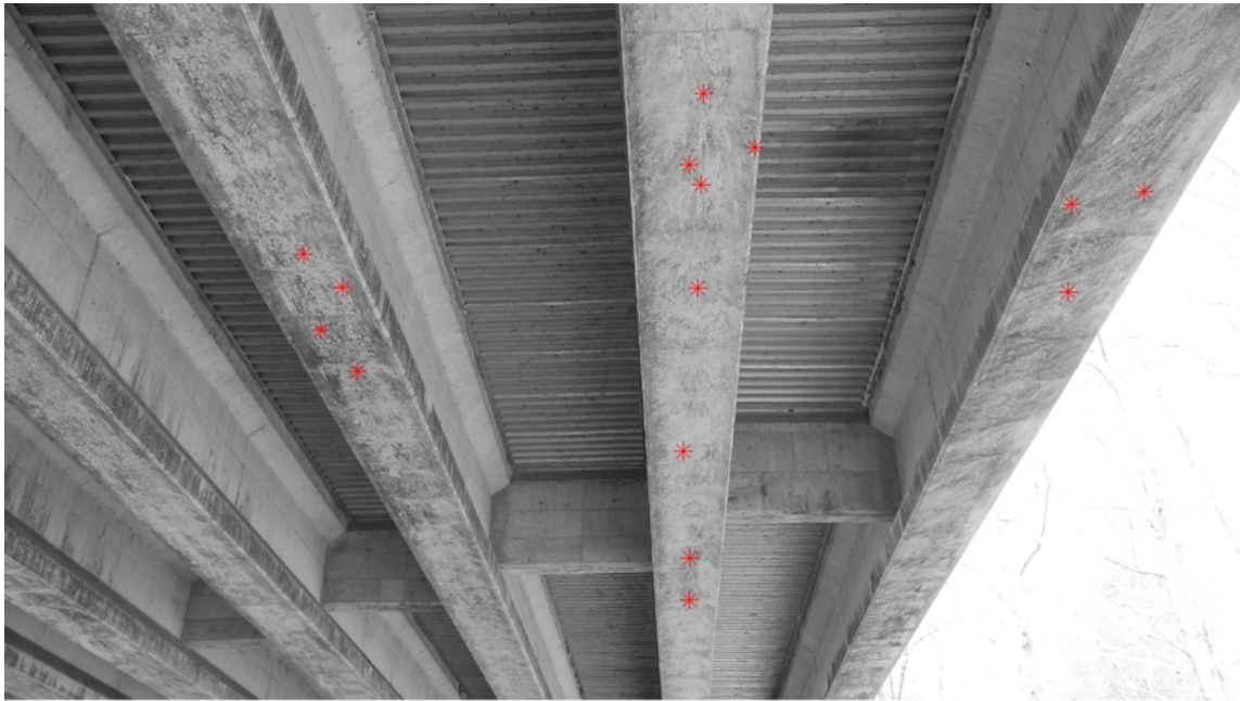
Figure 7.8. R CNN detection of beam flange: Example 1.
