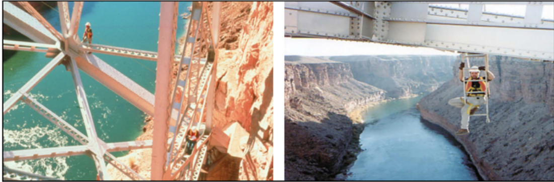
Figure 1.3. Bridge inspection team members inspecting tall structures (FHWA, 2012).
