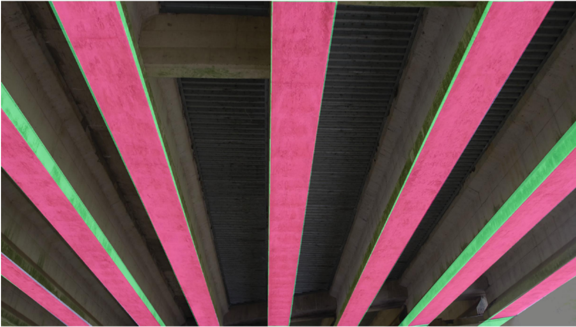
Figure 7.15. Full beam detection of beam flange: Example 4.
