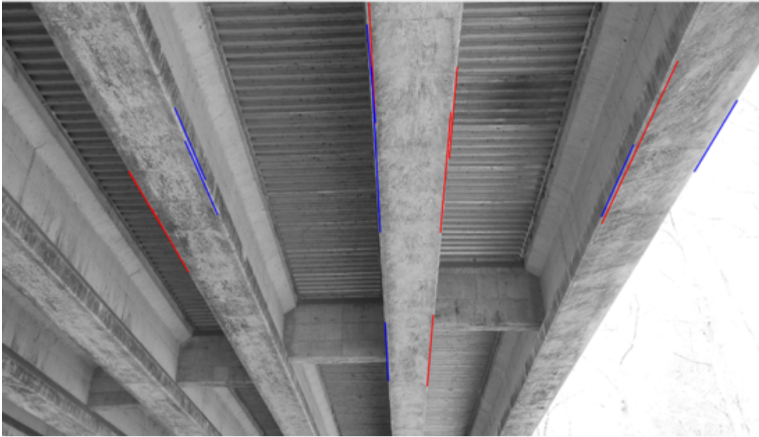
Figure 5.6. Example of proposed beam flange edges from all pROI detected in the image.
