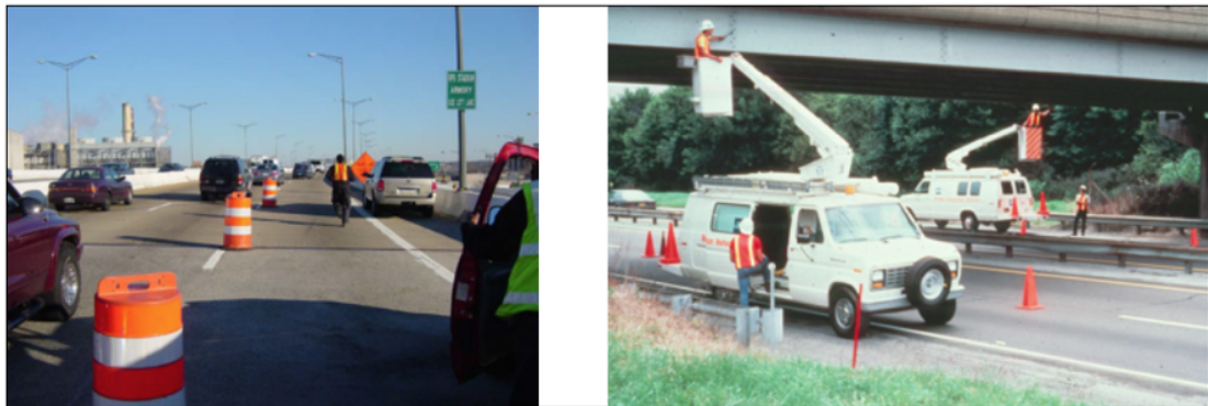
Figure 1.4. Bridge inspection team implementing a traffic control plan (FHWA, 2012).
