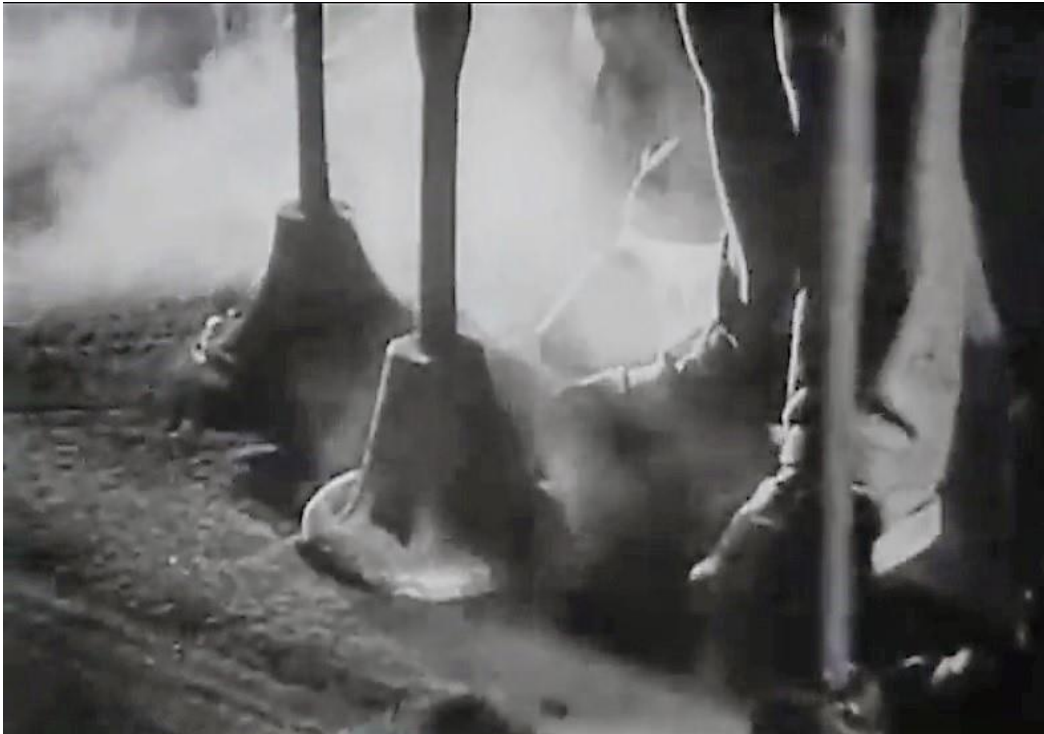
Fig. III-9. A shot of paving hot asphalt at the beginning of Asphalt .
