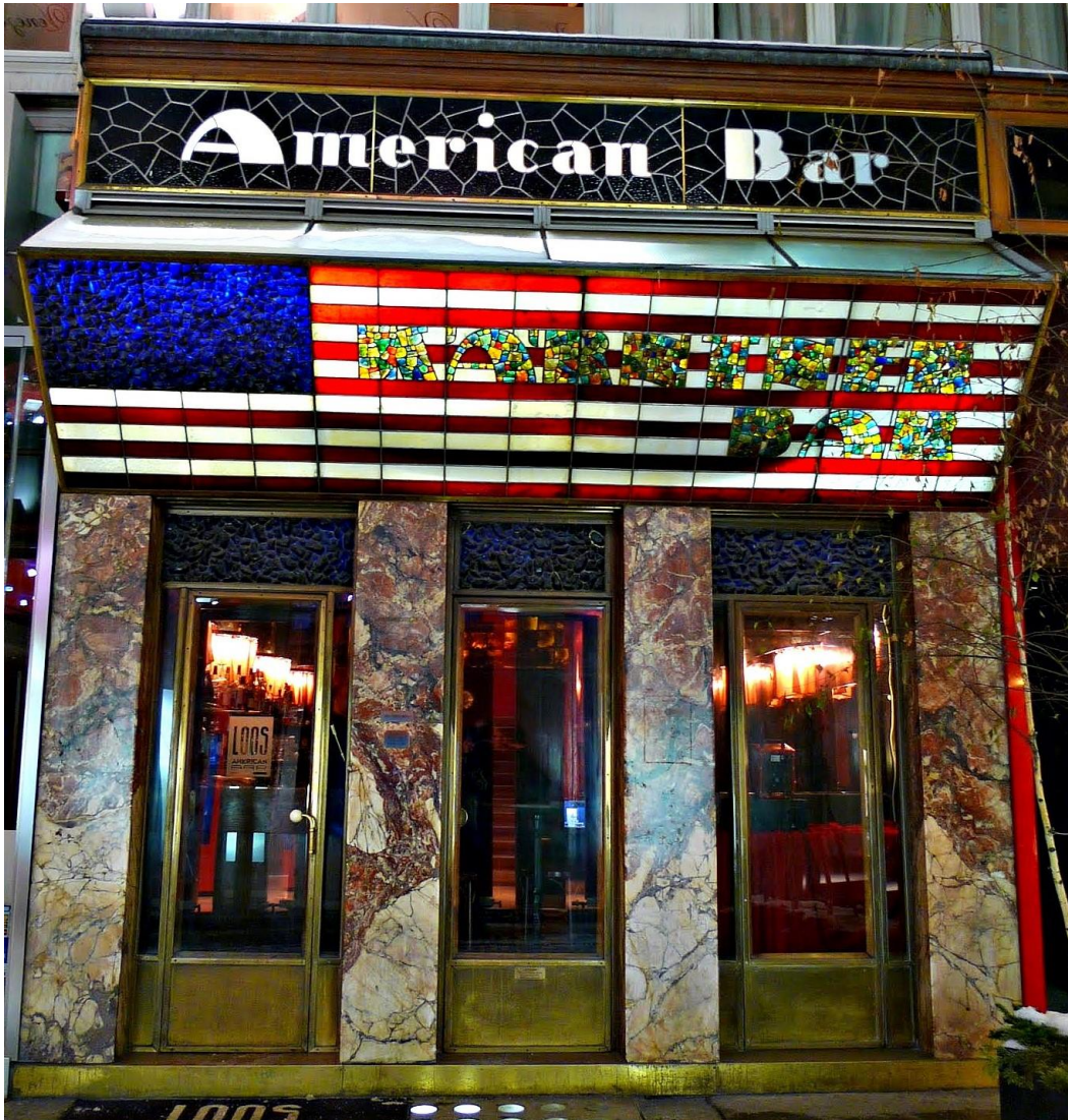
Fig. III-3. The facade of Kärntner Bar, also known as American Bar, designed by Adolf Loos.
