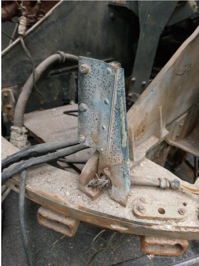
Figure N.7- Light blue paint is peeling, but obvious on a section of the tail turret. Little corrosion appears on these cast aluminum and steel parts, although the steel parts have faint rust marks in some areas. Photo by the author.
