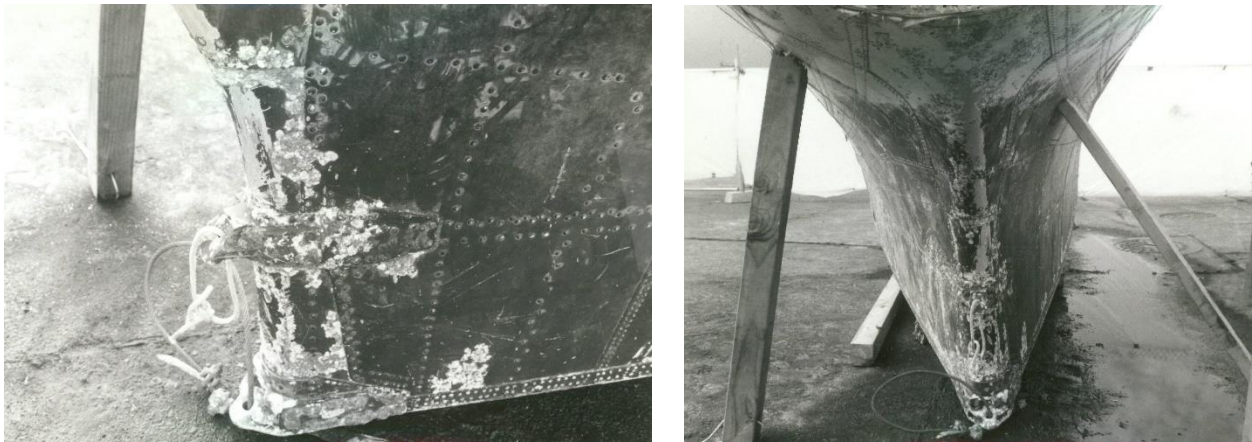
Figure 9.34- Corrosion nodules on the rear afterbody of the PBM-5 hull the day of recovery in 1996. Photos courtesy of NHHC UAB.
