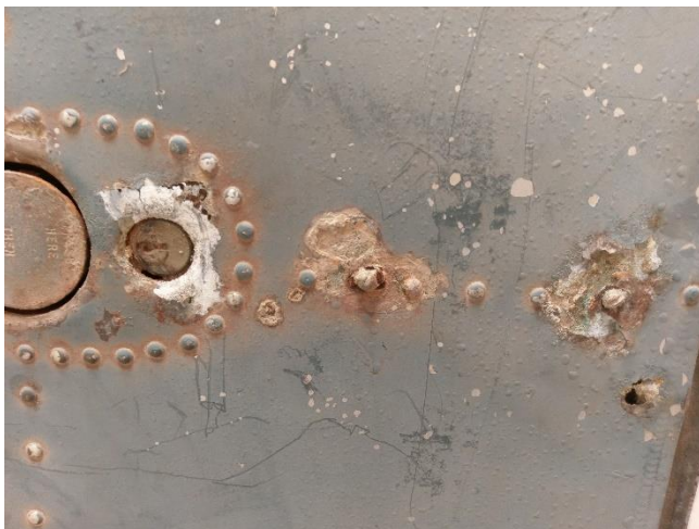
Figure N.8- A close-up of the pitting and exfoliation corrosion on the hatch door artifact recovered in 1980-1981. Blue paint still appears mostly intact. Photo by the author.
