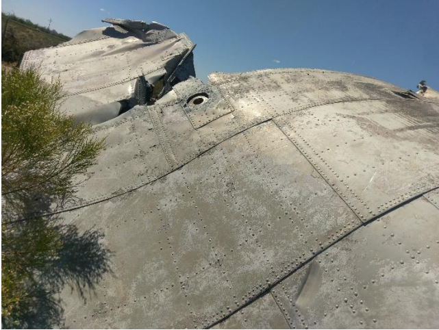
Figure N.15- The bleached bare metal side of the rear fuselage of the PBM-5, presenting with patches of light corrosion and increased corrosion around the circular hole central top of the photo. Photo by the author.
