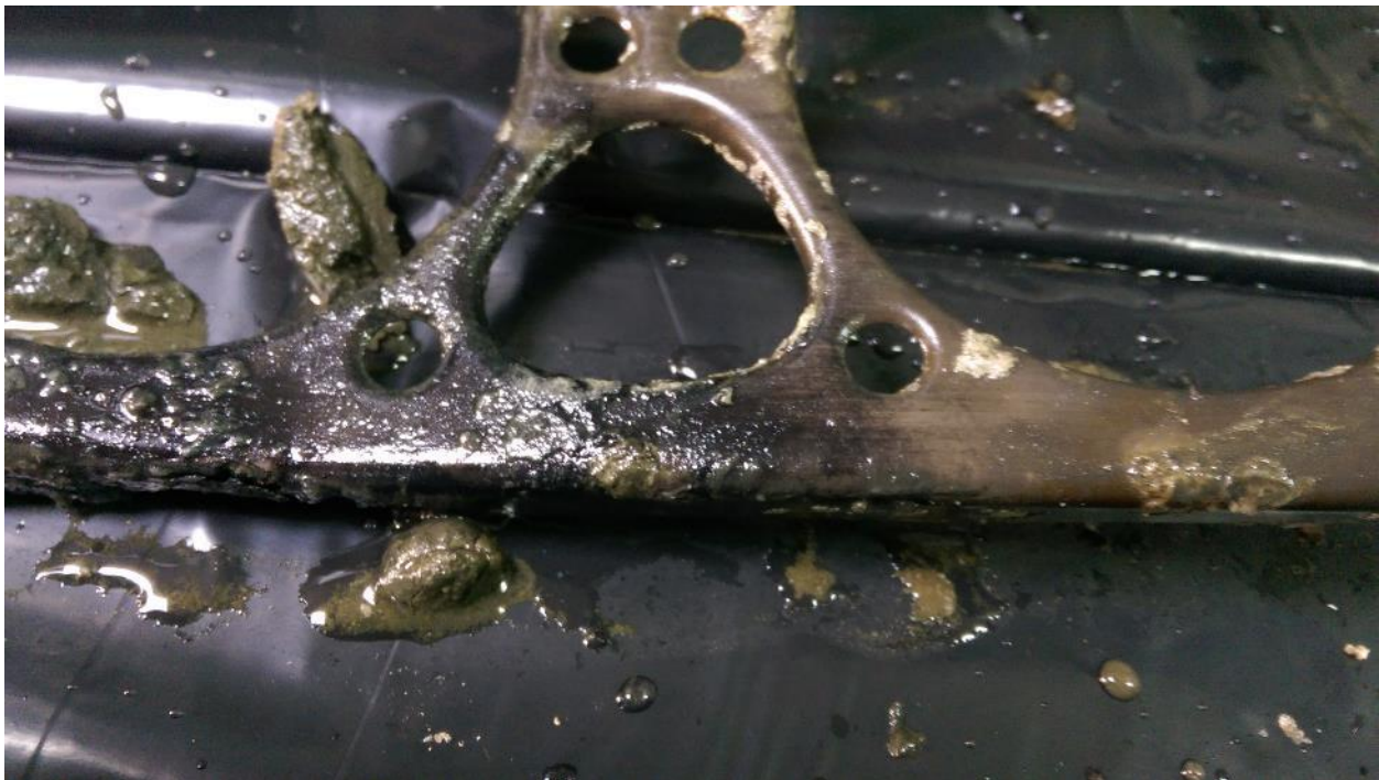
Figure 8.43- The demarcation line between the portion of the frame that was buried in sediment (L) and the side in the water column (R). Some pitted areas presented with black, maroon, and green corrosion products. Photo by the author.
