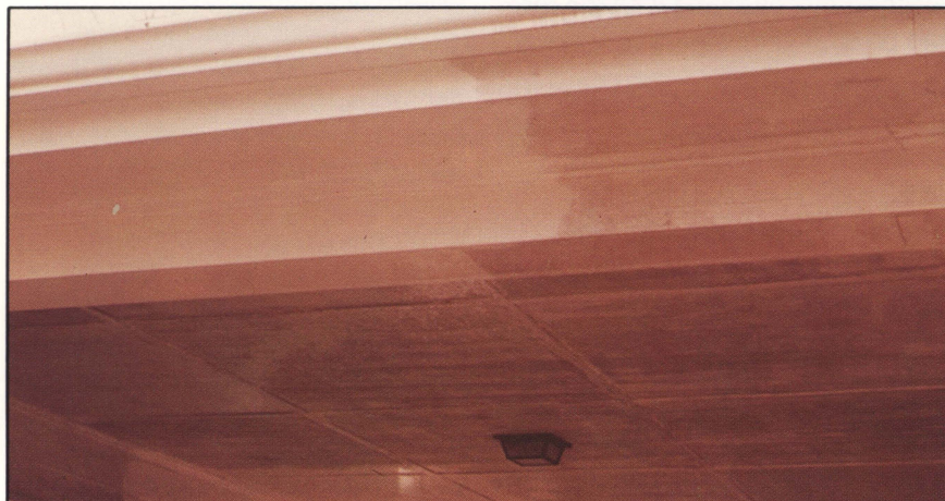
Mildew must be removed prior to painting. Painting over it, as shown here, will only hide it for a short time.
